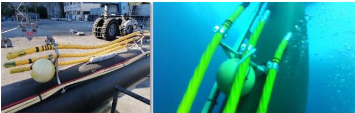
Figure 13 - RISE cables with 3 different painting configurations installed on the Western Mediterranean Sea Regional Facility spar buoy
